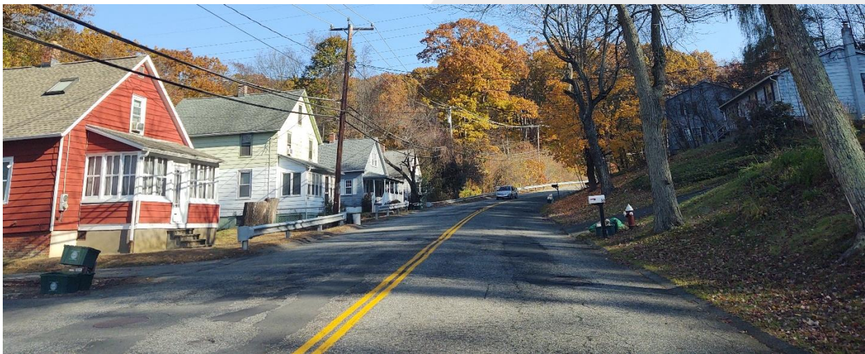
Ludlow Road at House #40 Looking East to Horizontal Curve
