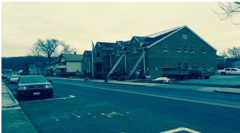
As is depicted, we only had the vapor barrier applied to the front of the roof, as it is where we were experiencing the leaking, the sun hits the back and we do not have the ice dam problems. This project may slightly exceed the \$15,000, the roofing quote came in around \$11K , but when the roof was stripped it was discover the soffit was not extended properly so I had it repaired and there will be an added expense of around \$4,000. It made sense to do it now not later.
