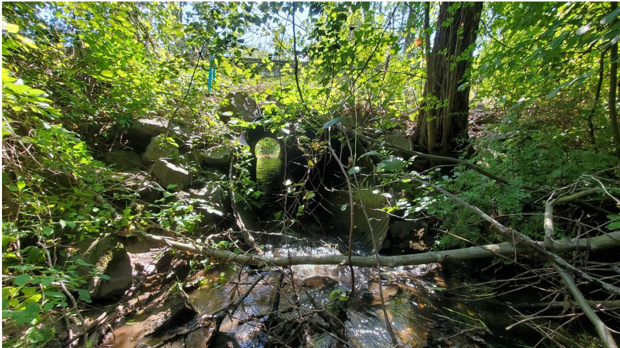
Photo 5. A reach of Elmer Brook, located approximately 10 feet upstream of the crossing at Pearl Street; the culvert inlet is at center. Looking south (downstream) near flag C314.
