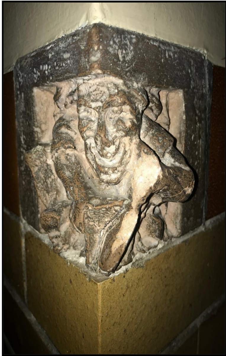
Example of carved "grotesque" located at numerous locations in classroom corridors.
