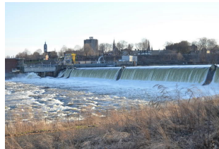
Holyoke Dam between South Hadley and Holyoke, MA
