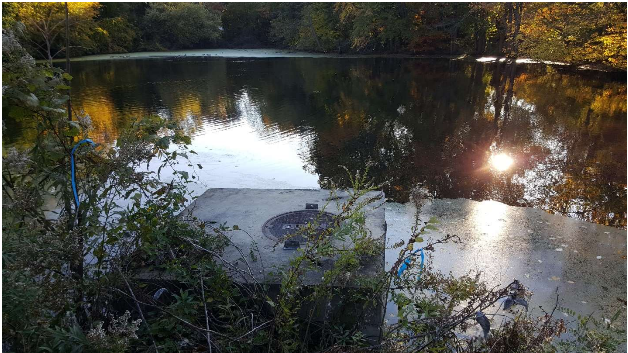
Figure 1. Titus Pond, with the inlet control structure to Buttery Brook in the foreground. Looking east-northeast near flag A101.
