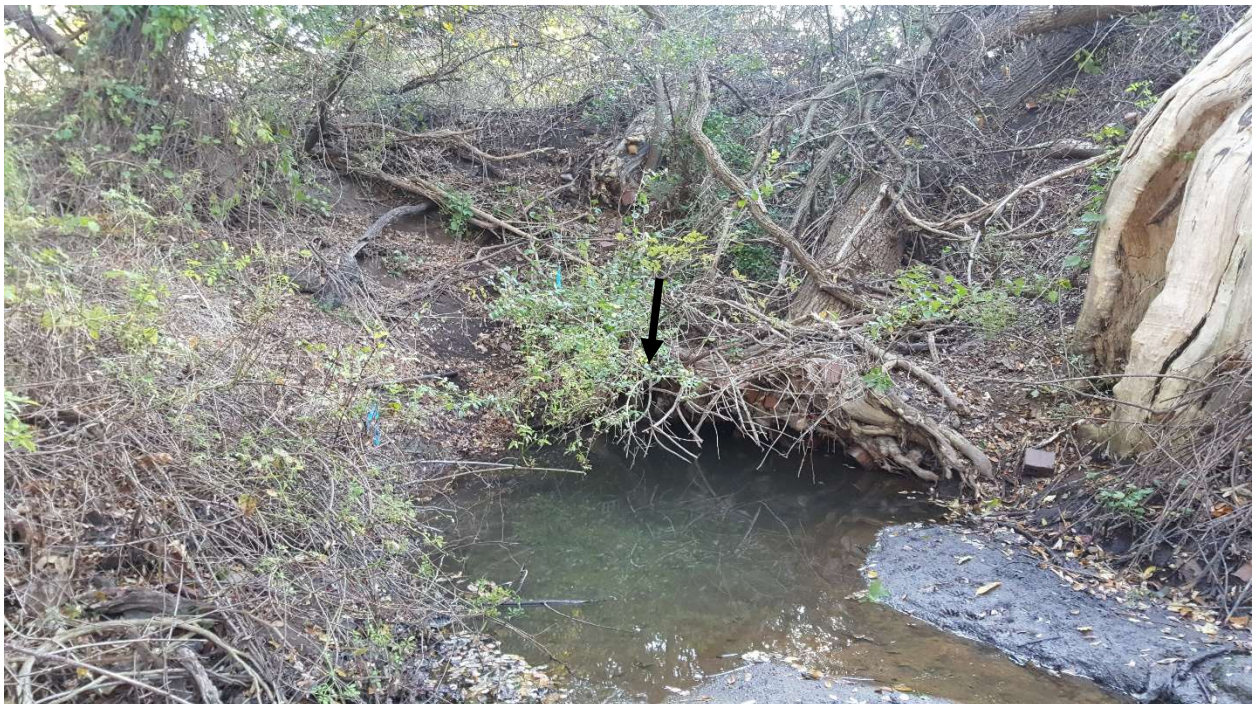
Figure 24. Outlet for Buttery Brook (flag series G700-G7-6 and H800-H812) south of Joffre Avenue. Outlet was almost entirely submerged and partially full of sediment. Looking east (upstream) near flag G702.
